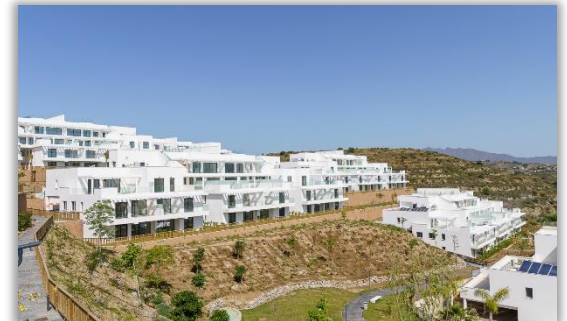
Casa Banderas | 200 units Malaga 2019-2020
